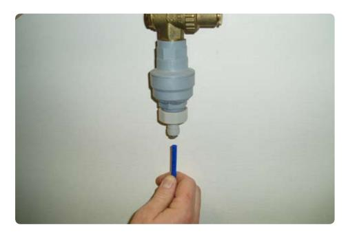
**Step 5;** Push the flexi-pipe through the hole in the back of the machine.
