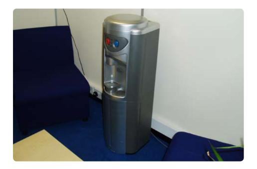
**Step 10,** Replace the front cover and position the machine where desired. Once in place, empty half a bucket through the dispenser taps, and turn on the power. NOTE: PLEASE ENSURE WATER IS PRESENT AT THE HOT TAP BEFORE SWITCHING ON THE POWER.
