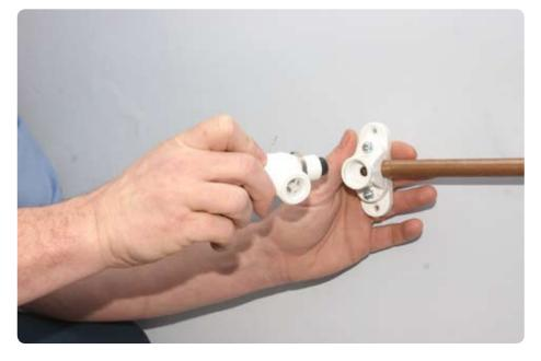
**Step 3**, once the tap has been screwed in as far as it goes, tighten up the locking nut.
