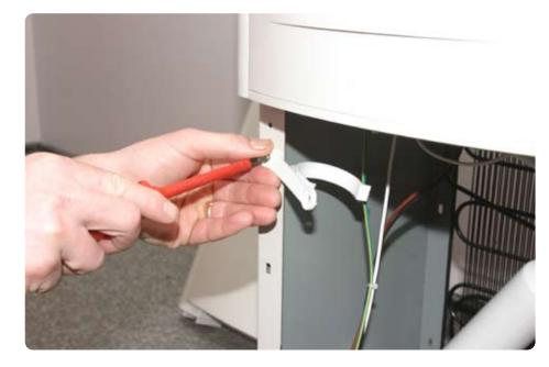
**Step 7,** Push the flexi-pipe through the hole in the back of the machine. Connect the flexi-pipe (which connects into the inlet fitting) into the top of the filter and turn on the water at the washing machine valve.
