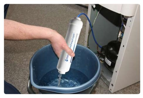
**Step 9,** Connect the tank filler pipe into the other end of the filter and place in the bracket.
