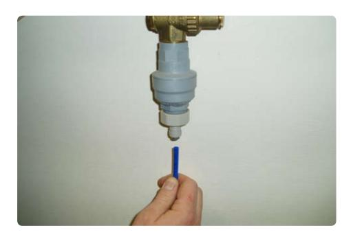
**Step 4**; Push in the grey connector into the back of the machine.
