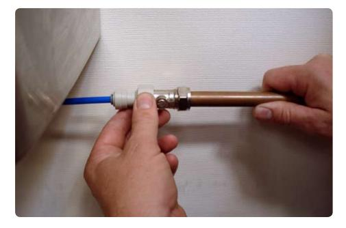
**Step 5;** Attach the drinking water supply to the bubbler head using the blue flexi pipe and connector.
