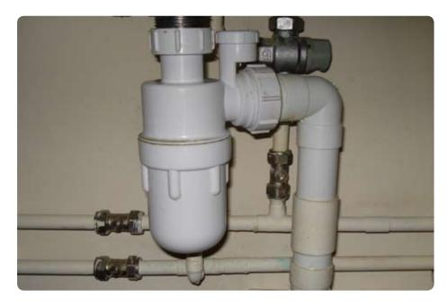
**Step 7;** Turn on water and check for leaks.
